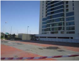
Picture-4 Fire-affected Car Park in front of Tamweel Tower.
