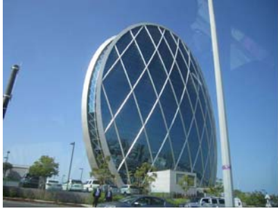
Picture-5 Example of Alpolic Sandwich Panels Used as Exterior Façade Frame of Aldar Headquarters Building in Abu Dhabi.
