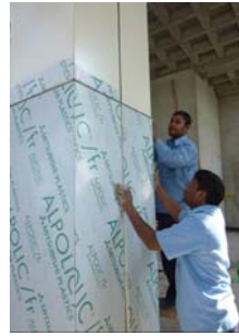
Picture-6 Construction-site in Dubai, Installation of Alpolic sandwich panels.
