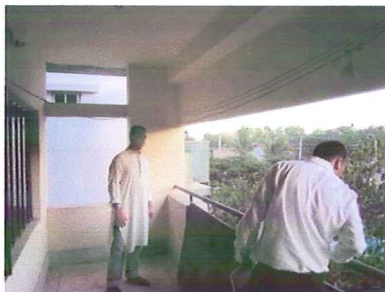
Picture-8 At balcony on the Second floor.
