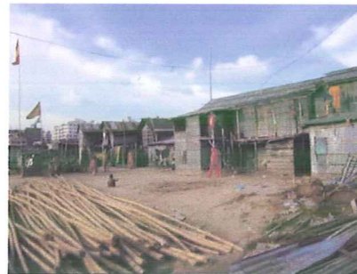
Picture-11 Bamboo construction in Dhaka
