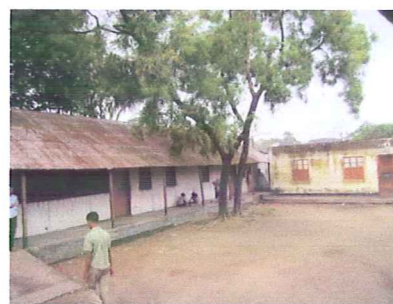
Picture-5 Playground and fire-affected buildings of UCEP school.
